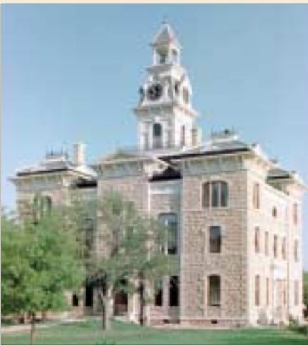
The Shackelford County Courthouse, Albany
