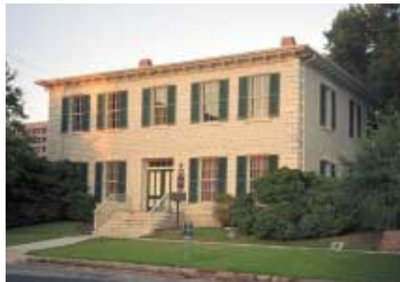
The THC's executive offices are located in the Carrington-Covert House in Austin.
