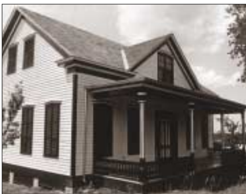
Above: The Thomas Kraitchar, Jr. House, funded under the Texas Historic Preservation Program, in Burleson County is shown before (top) and after renovations.
