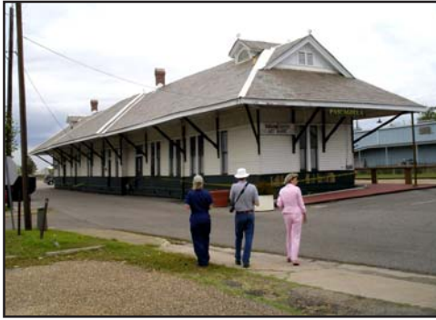
L&N Depot, Southeast Elevation
