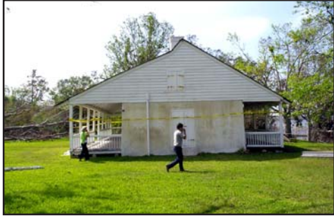
Old Spanish Fort, East Elevation
