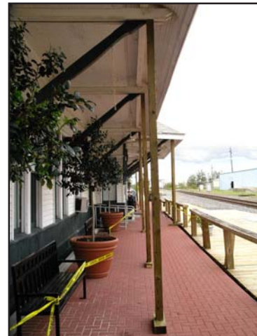
L&N Depot, shored brackets
